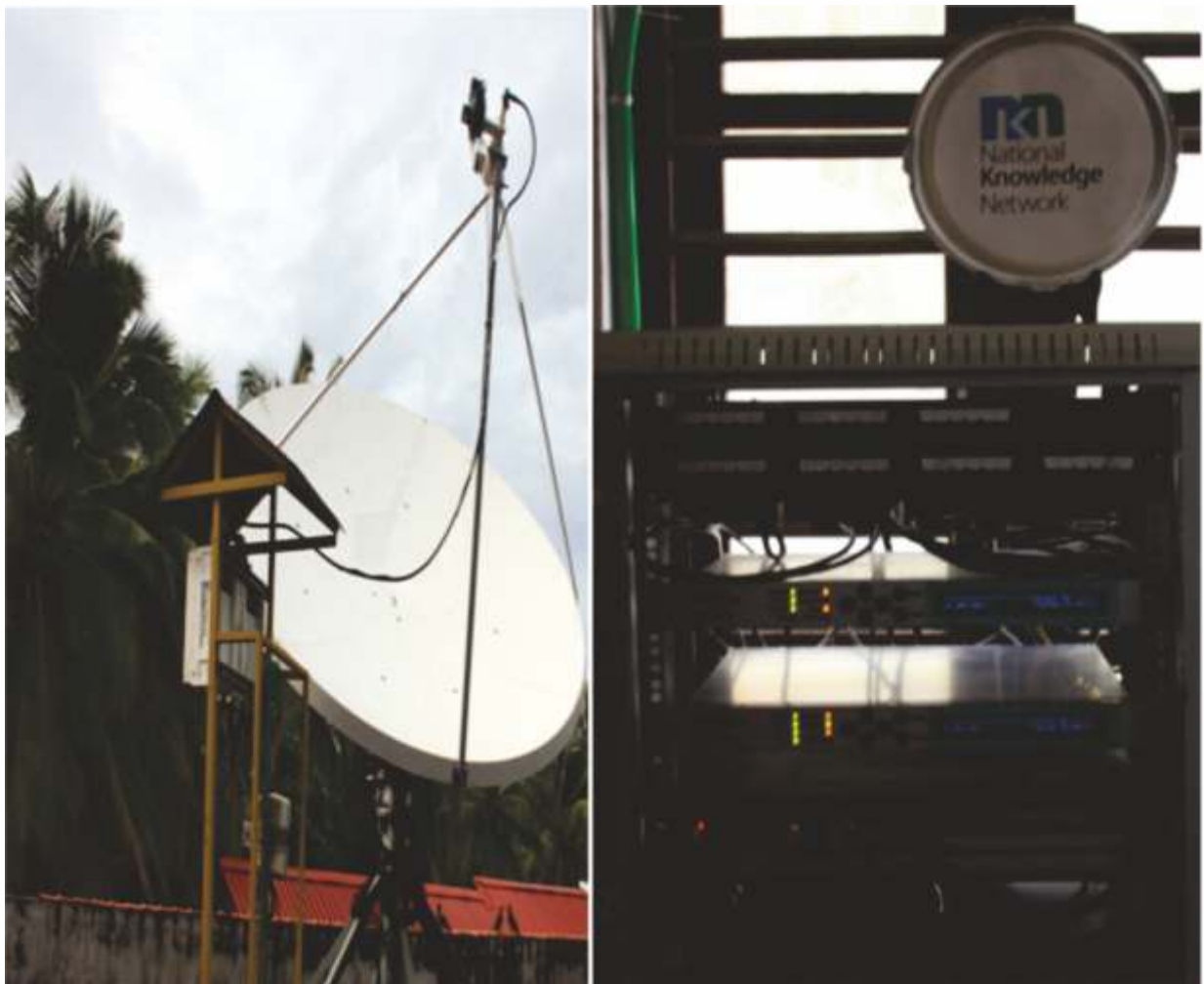
Fig 20 : High Capacity SCPC VSAT at Kavaratti, the U.T. of Lakshadweep Island for NKN Project
