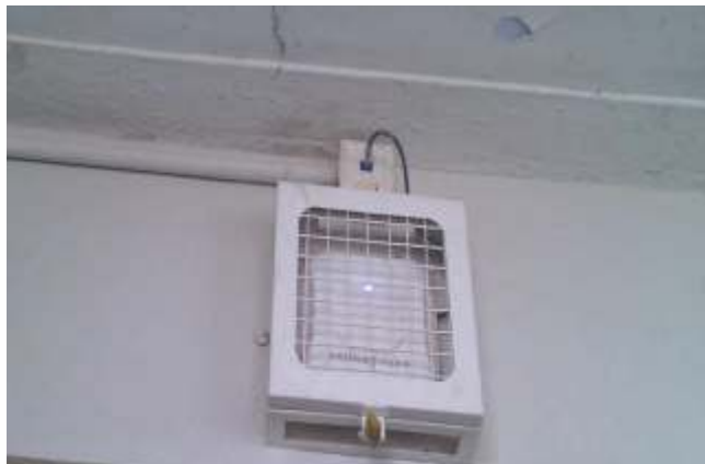
Fig 28 : Wi-Fi Access Point at SPPU, Pune with protective cage
